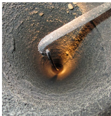
Lower flue wall, soot evenly spread, grey colour, 28 July
