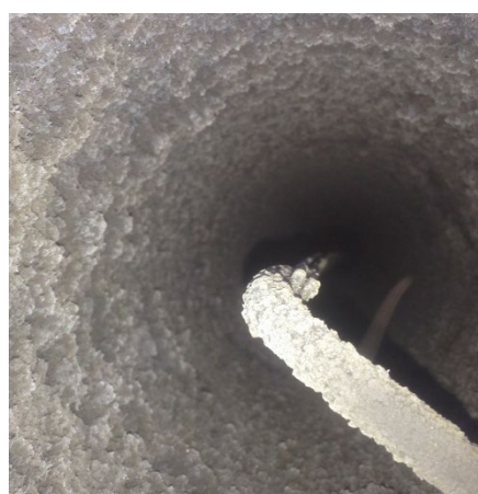
Light grey dust, approx. 5-8mm evenly spread on lower flue wall, 3 September
