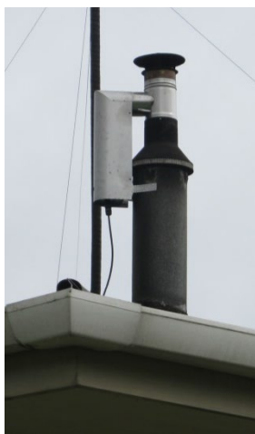
OekoTube circuit box on chimney
