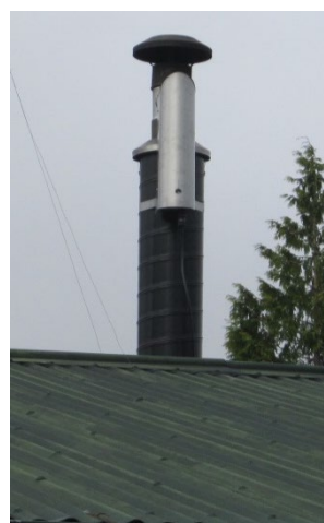
OekoTube circuit box on chimney
